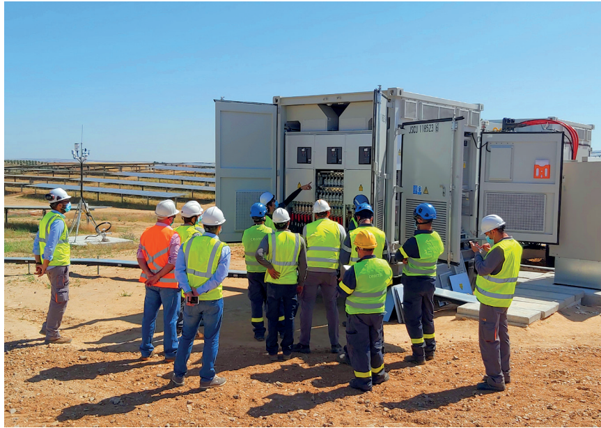
Sungrow experts providing a customer training on site
